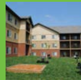
The Crest at Baker Creek; newly constructed multi-family units on the east side of Des Moines.
